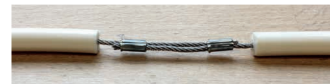
1. Join exposed reinforcement with press sleeves
